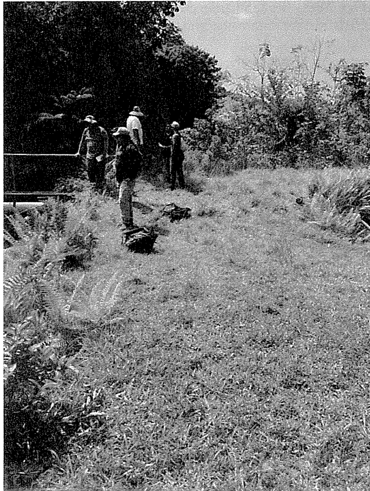
Figure 7. Location where stream will cross access road.
