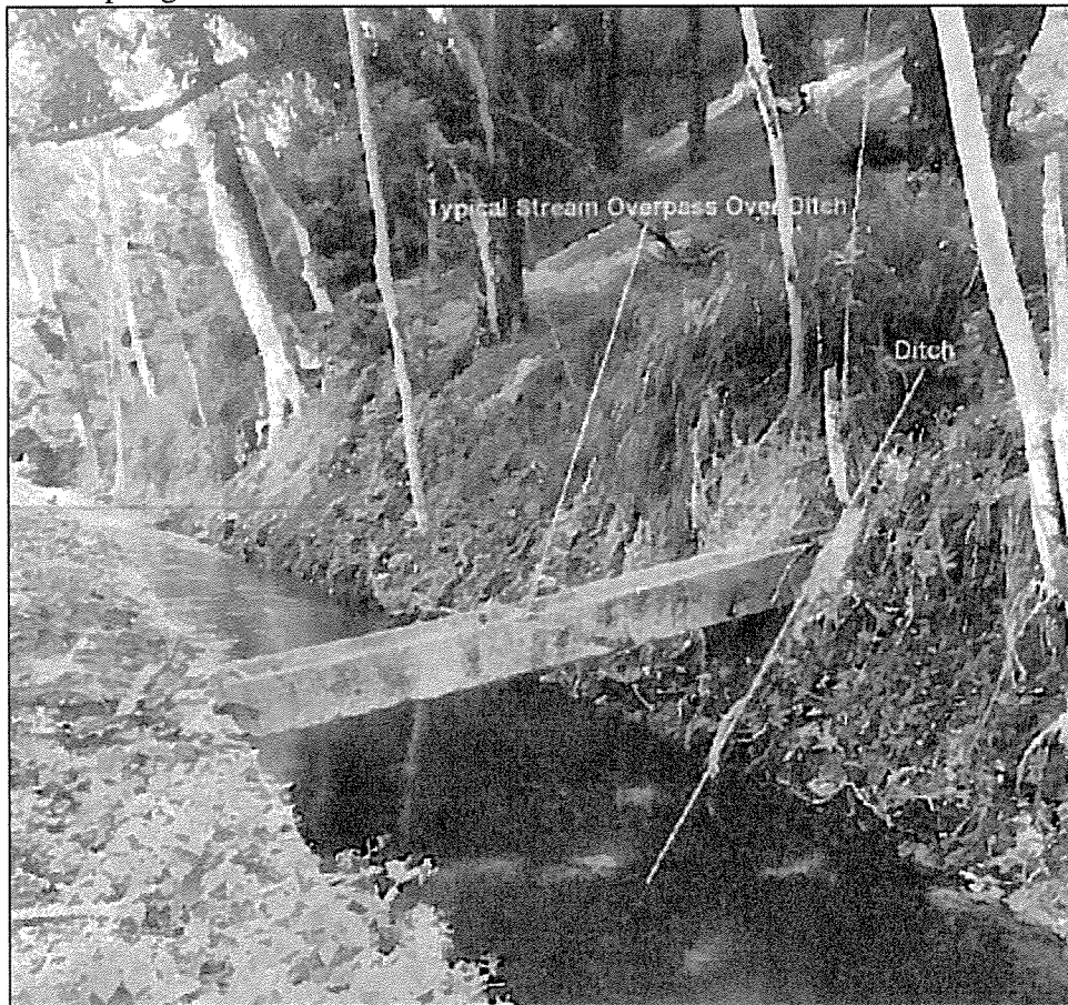
Photo 3. Typical “stream overpass” intended to prevent the ditch from intercepting a stream.
