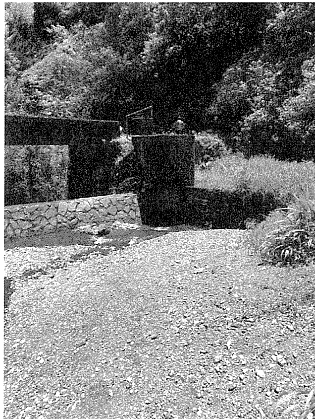
Figure 11. Dam, gate, and control structure at K-21.
