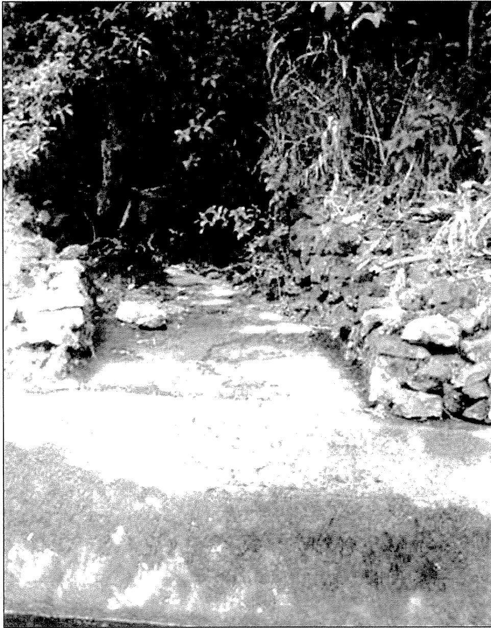
Photo 12. Hauolowahine runoff pad at Koolau Ditch (K-30d).
