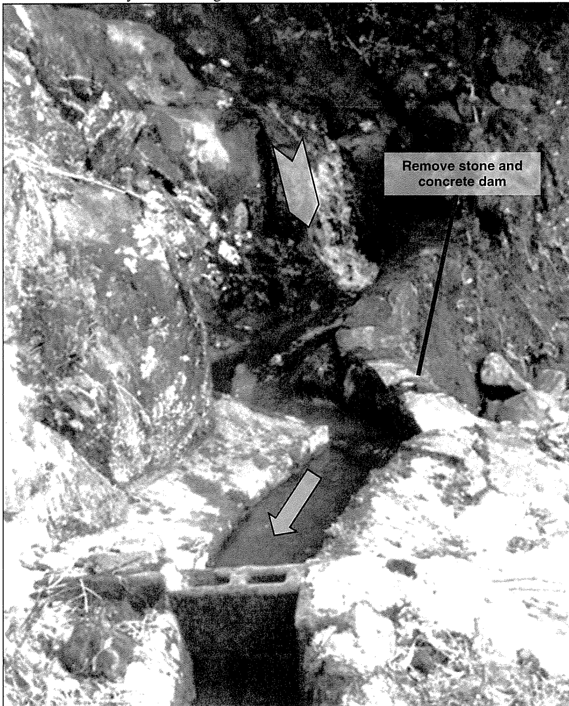
Photo 11. Tributary flows through concrete lined ditch (EMI, 1989) (K-30b).
